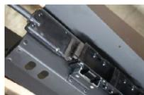
The infeed snaps into the power block of the first technology center. The power blocks come pre-installed in the technology centers from the factory. There are four connection points on each power block, this allows for the infeed and jumpers to daisy chain multiple power blocks.
